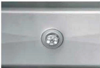
≡ Photo 15: centralised drain
